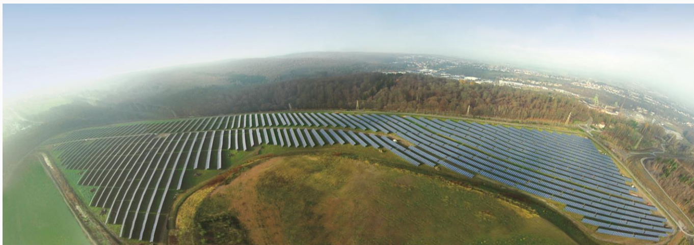
Ground-Mounted Smart PV Plant, 10MW, Krempendorf, Germany
