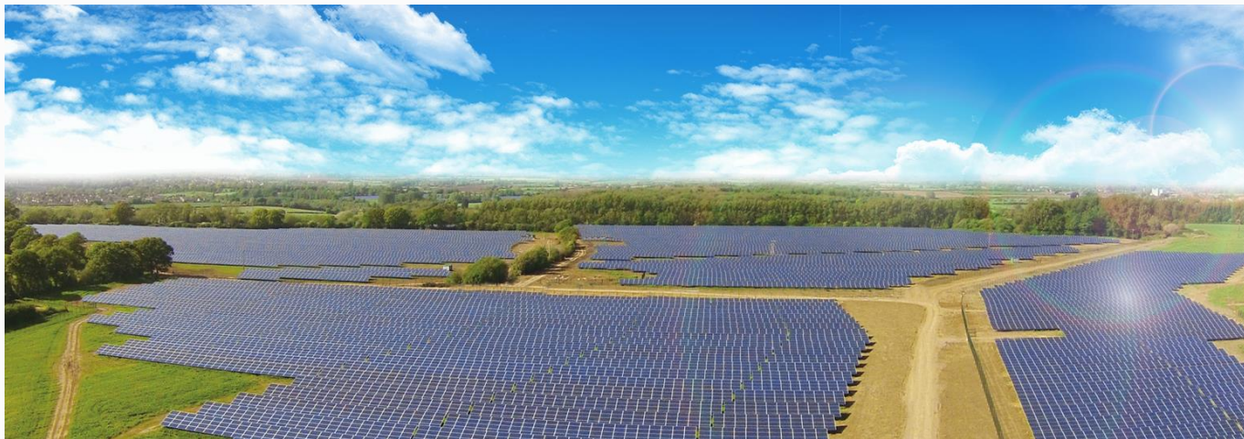
Ground-Mounted Smart PV Plant, 13.5MW, Melksham, Wiltshire, UK
